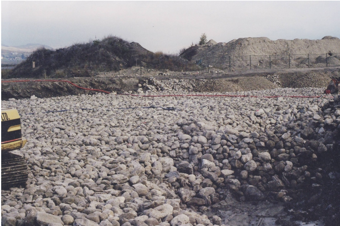
Figure 7 Backfilling the Foundation Excavation
